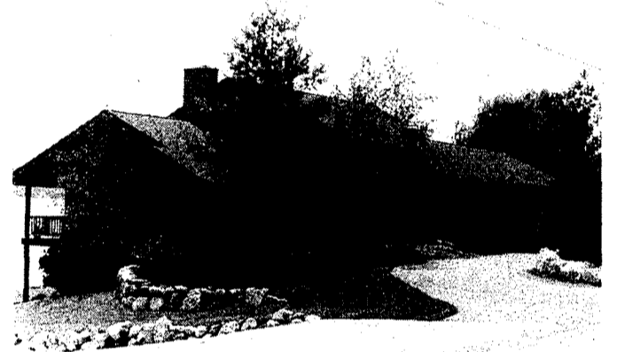
The Michael Gabos home on Michigan Avenue is the residential recipient of the annual Marv Loding Awards. The Loding awards are now a center of controversy since a Boyne City Commissioner asked that the Planners who recommend the awards, develop a criteria based on pride in civic matters as well as beautiful grounds.
