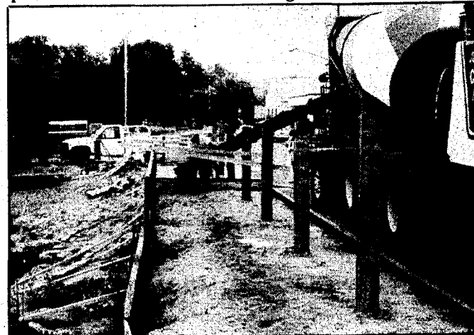
With the walkway over the bridge all formed up, workers started pouring the cement Tuesday with the intention the walkway will be ready for the weekend activities.
