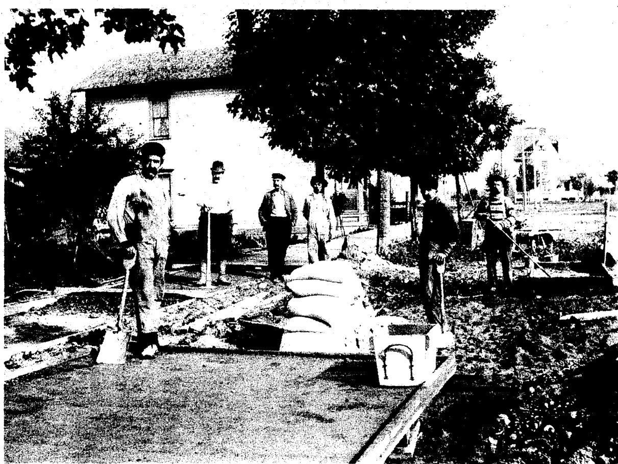
It was interesting, the way workers in the old days installed the sidewalks. This crew, which included Jayson Lewis, the grandfather of Thelma Behling, put in some of the first sidewalks in Boyne City sometime in the early 1910s. The street was Water Street looking east. If you were to locate where the picture was taken, it looks like it was about in front of the store Country Now
