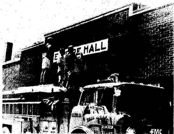
Freshening up the fire hall in East Jordan recently, volunteers from the department spent some time over the recent weekend to apply some paint to the nameplate of the building located on Main Street in East Jordan. Using a fire truck for a scaffold, were those painters and helpers. The truck was kept running in case there was a fire and they have to move it out of the way of the other fire trucks in the building.
