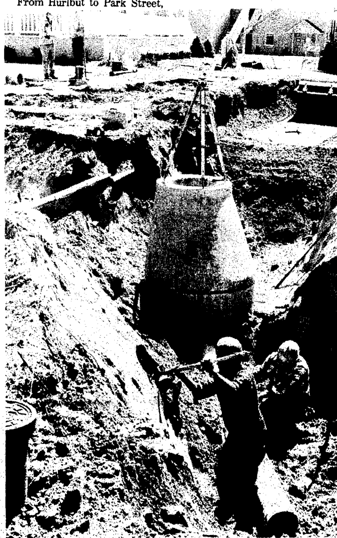
Workers spent two days working at the intersection of East and State Streets, getting all of the underground work done before the paving can begin. The work is part of the rebuilding project of M-75.
