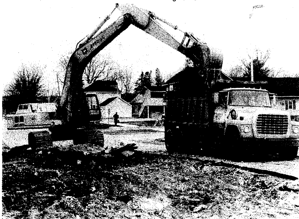
Work has started on the rebuilding of M-75 as crews down for long periods of time. This section, East Street, is the first part to be completed. Next will come Water Street and Boyne Avenue. Completion for the job will be 100 days from Monday barring rain days.
