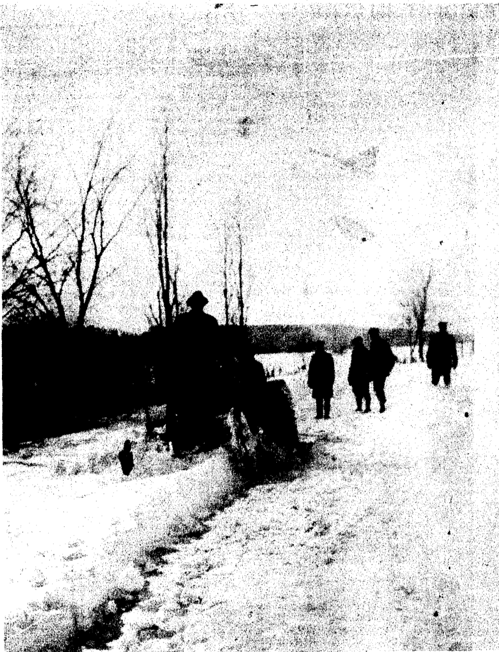
Early attempts to move snow out of the way created this tractor with steel wheels, back in the twenties, for the Charlevoix County Road Commission. The tractor slowly worked its way down
