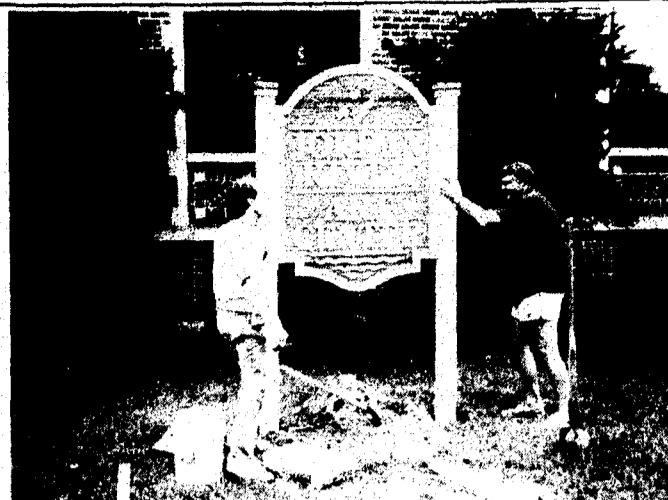
With the installation of a new sign, Jordan River Art Center officially opened with a grand opening reception Saturday, June 30. Installing the sign are Jordan River Arts Council member Jack Bechtel (right) and Brian Oliver, employee of Boyne City's The Wood Shop.
