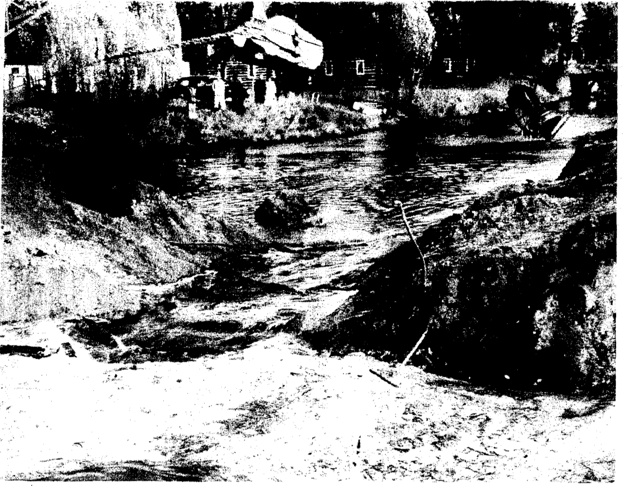
With the water rushing through the broken earthen dam, the water in the Boyne River started a new path to the lake as workers dug out the rest of the dam. The present path has been used for about 30 years as this work was done in the late fifties or early sixties. According to locals, the only thing bad about the
