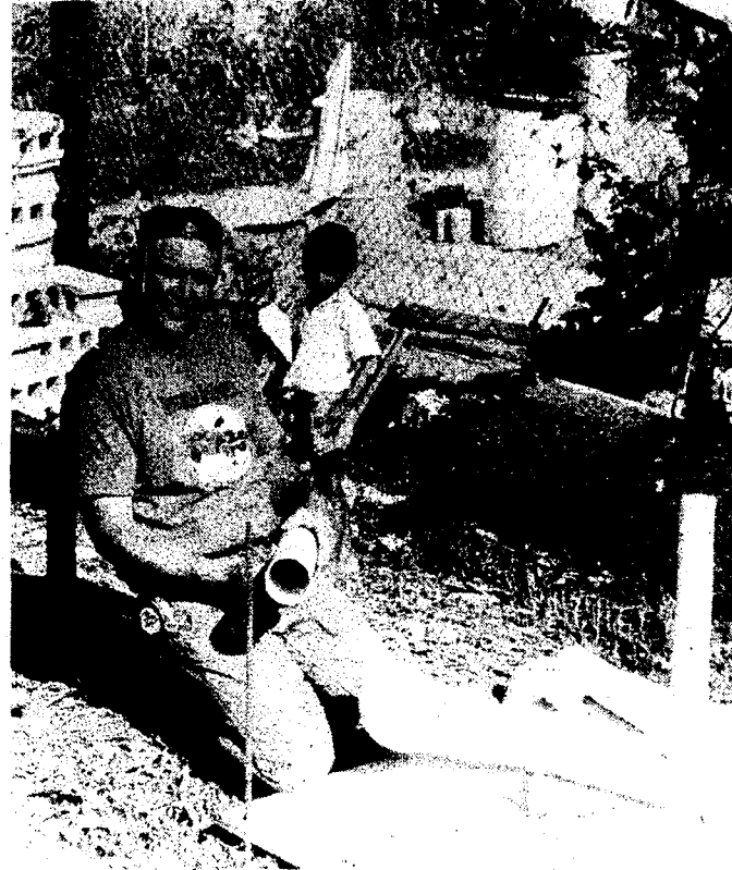
Nord Schroeder took a break from installing some plumbing pipes during one stop to replace a home while in Puerto Rico. Almost helping was this small boy whose mother owned the home that was destroyed by hurricane Hugo.
