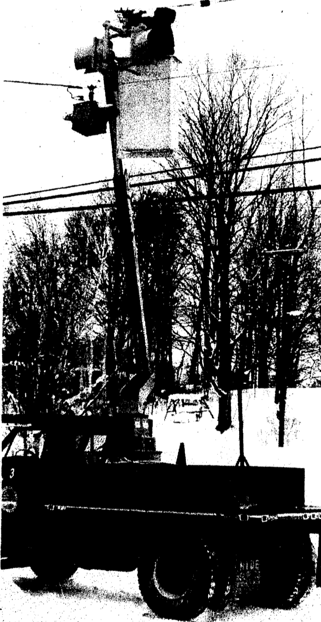
City workmen and electrician Joe Bower spent some of the holiday week installing a new blinker light warning drivers to slow down when they come to the intersection of Groveland, Lake and Michigan Avenues. The intersection has had numerous accidents in the past year and is one of the more dangerous intersections in Boyne City.
