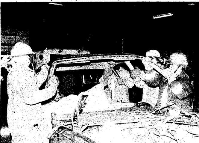
After instructors told the trainees that the car had to be opened up, members of the Melrose Rescue Squad used their equipment to cut off the top of the car to make it easier to get at the victims.
