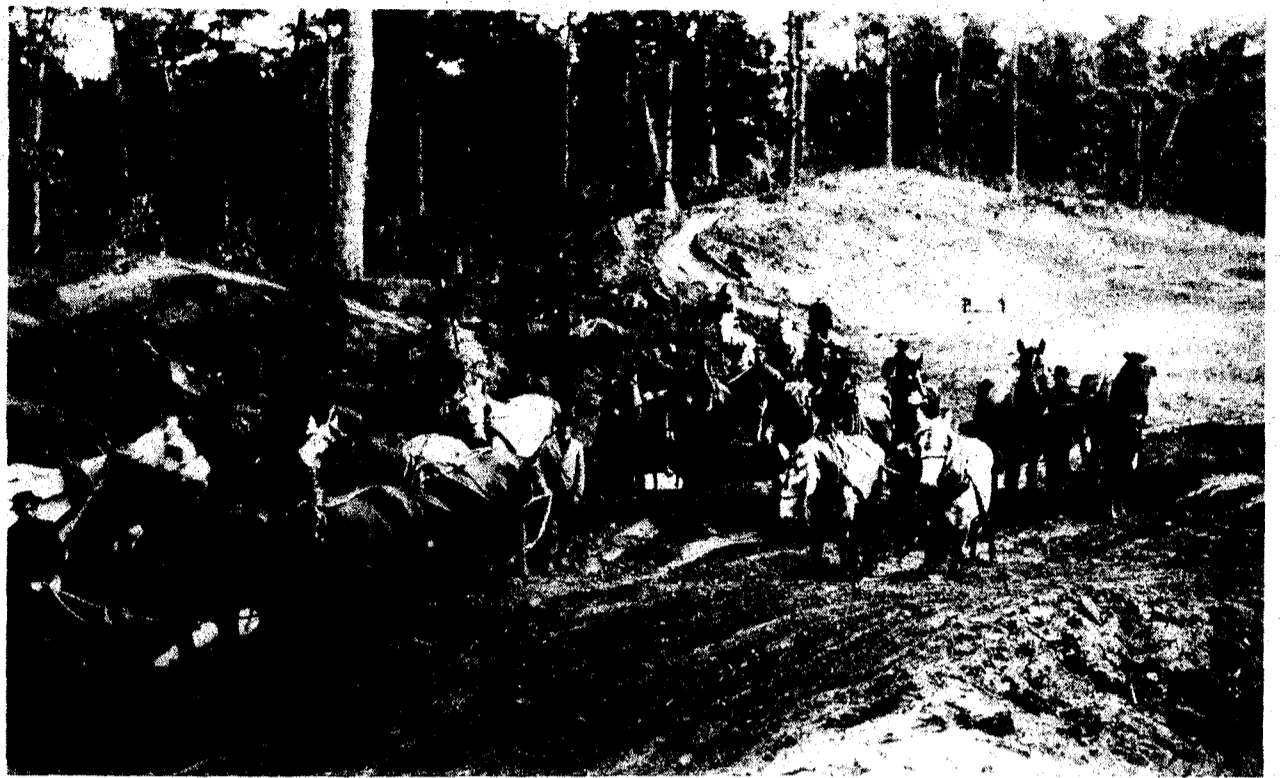
It took a lot of horses, and even more men to build the roadways for the trains back around the turn of the century. This picture shows some of the crew that worked to help build the right-of-way
