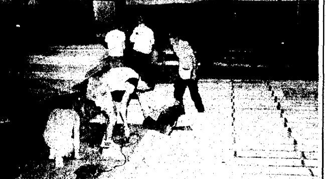
Every year, the dance floor is constructed from scratch by workers a few days before the event.
