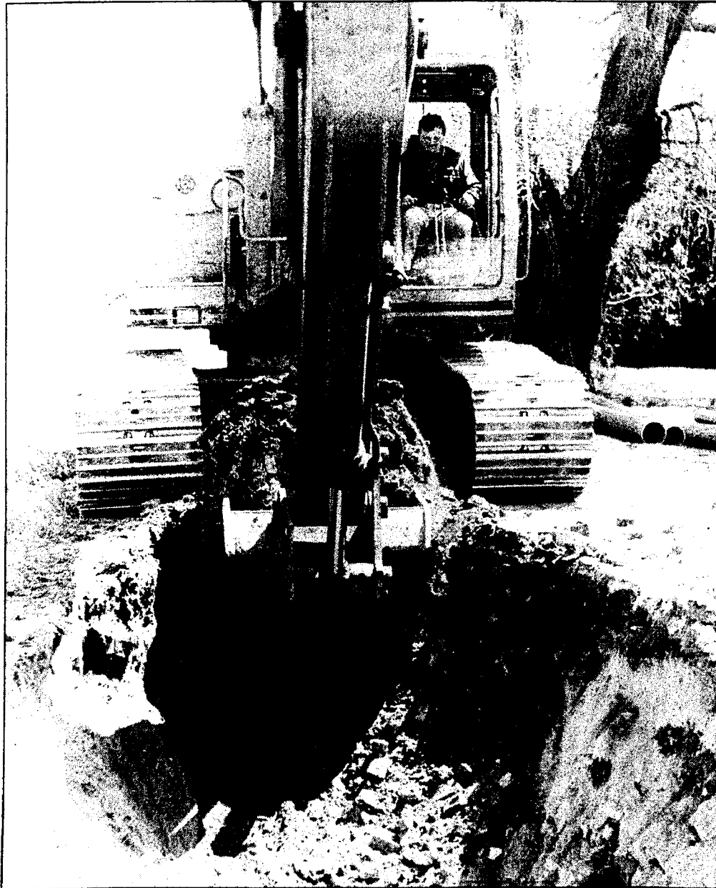
It must be the construction season as the diggers and dozers from C.H. Smith Company are out around town working on more of the infrastructure im-
