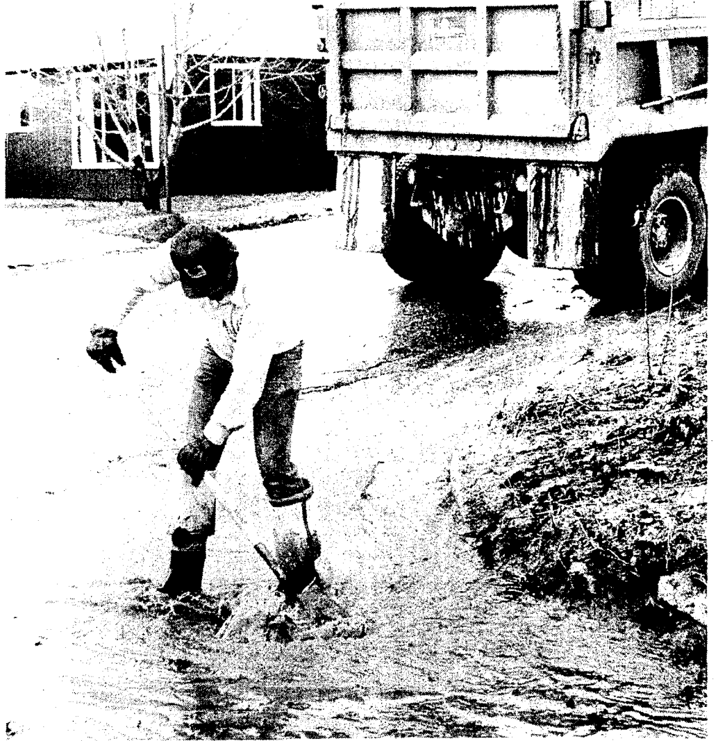
Keeping a catch basin clear of debris occupied the city worker Monday, as he tried to keep up with the melt-off of about two feet of snow due to the 70 degree weather Monday.
