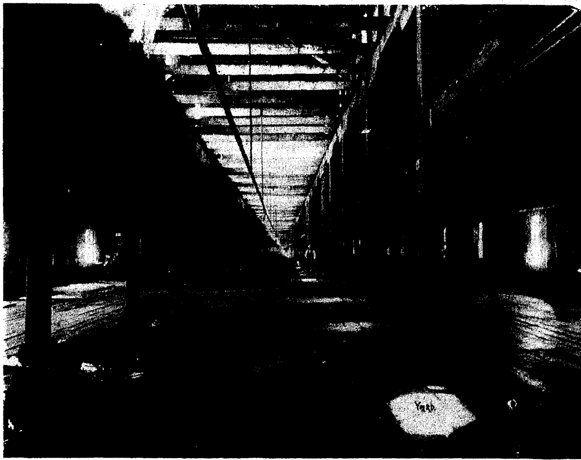
The "wet end." That is what they called this part of the former Boyne City Tannery back when they were producing tons of hides each day for shoe leather. Although it looks like the wet end was nothing but a room with a wood floor, the planks that made up the floor were removable and covered up the vats where the hides were soaked in different solutions getting them wet enough to accept the tannin that
