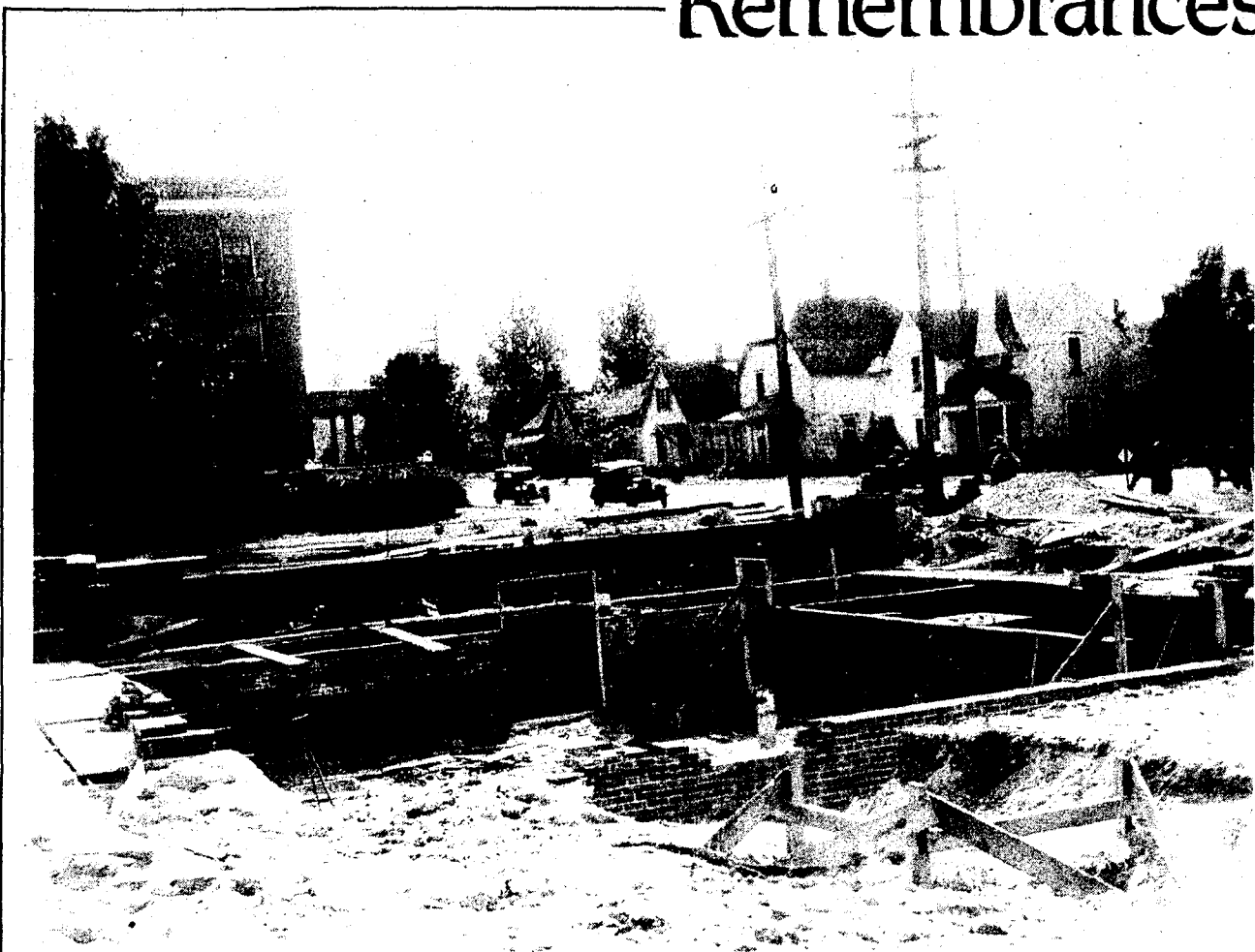
During the Great Depression, workers from the W.P.A. started building the present day Boyne City post office. This picture was taken from the back corner of the lot looking out at the intersection of East Street and Water Street. The project took several years to complete according to information on the photos provided to us by the Postmaster.
