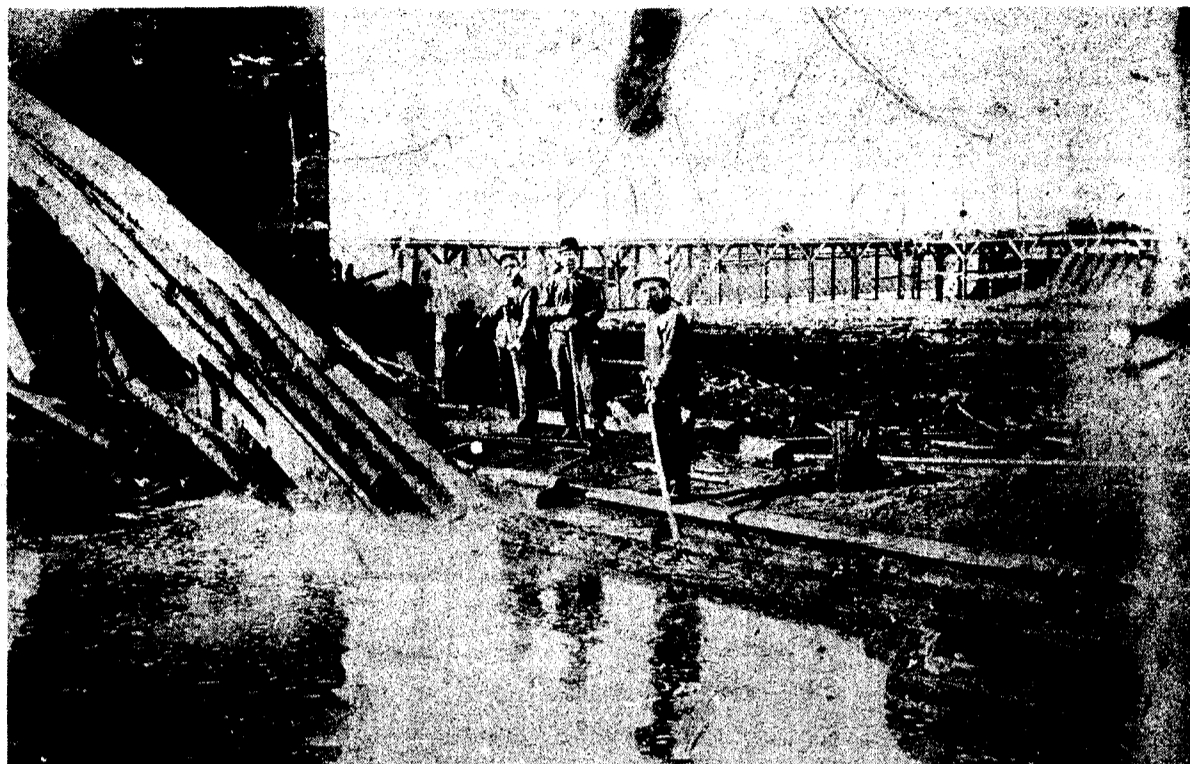
Come on, grab that ol' pike pole and help move these cedar logs into the conveyor so Mr. White can make shingles of them. This picture shows one of the ways the logs were moved around when they were brought to the mills. Workers with pike poles pushed, shoved and coerced the logs to the chute that would take them to the saws. This crew took a few moments out of a
