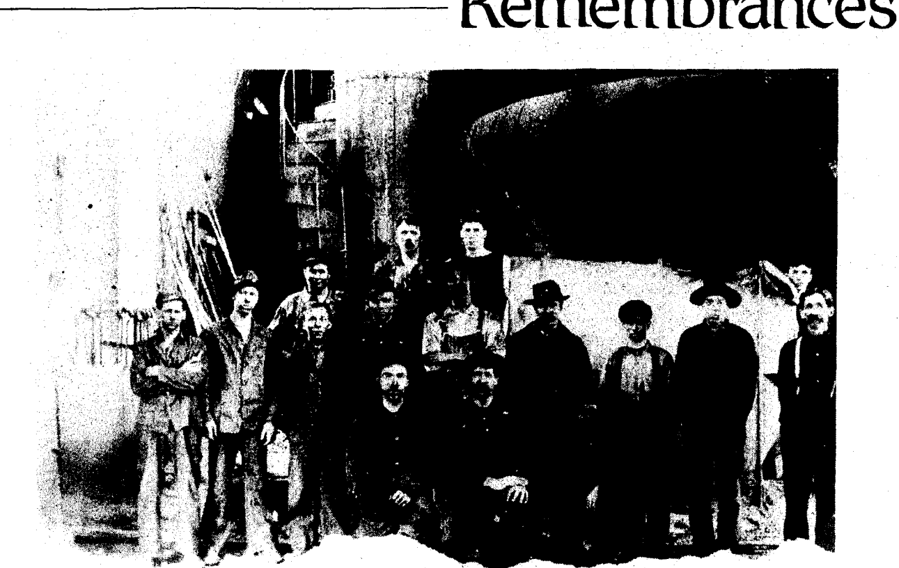
Members of the pouring crew of the former Boyne City pig iron plant took time out to pose for this picture. The crews would pour the molten iron into specially formed troughs in the sand floor. Some of the blast furnace can be seen in the
