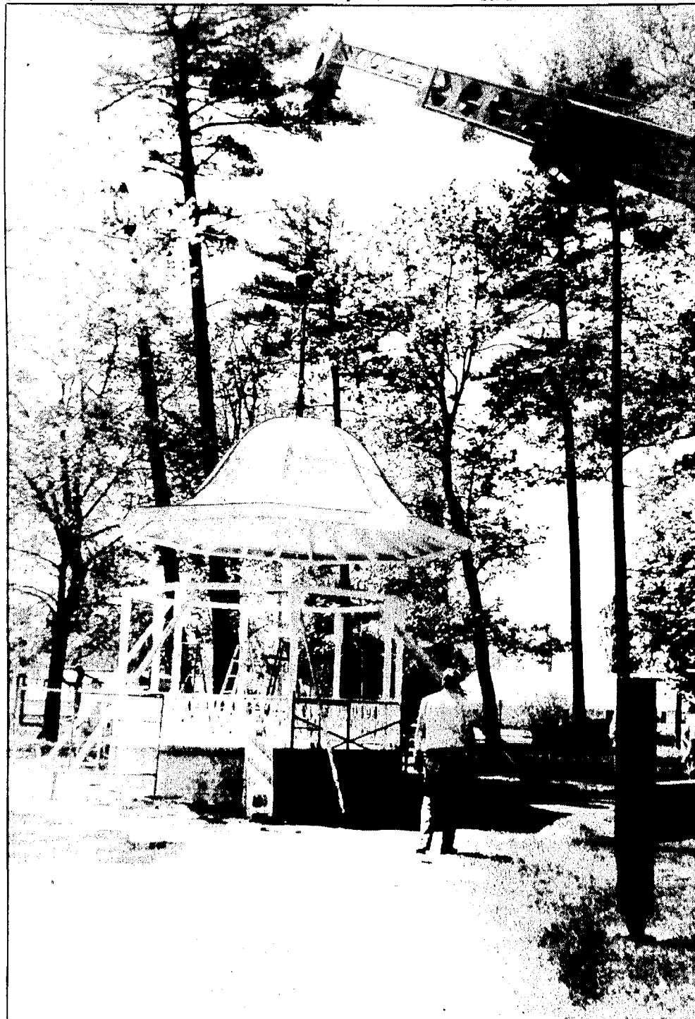
With the help of a big crane, the nice shining copper top of the new gazebo being constructed at the Old City Park in Boyne City was installed Monday. The gazebo was donated to the city by Gordon Flodquist
