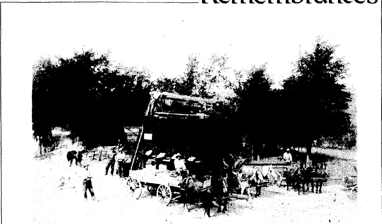
With all of the construction happening in Boyne City, we thought this picture of a gravel and stone separator back in the early times of the century was appropriate. This picture shows the machine in use with teams of horses and wagons getting filled up from the appropriate bin. Think how long the
