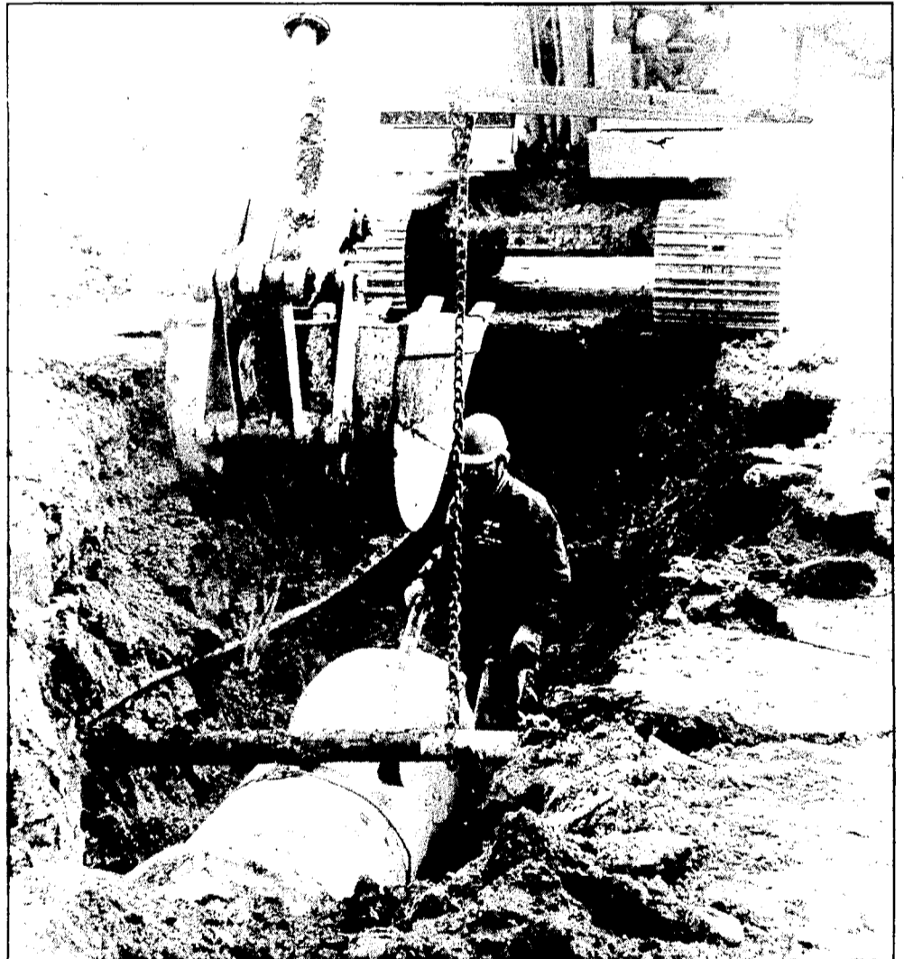
With the advent of spring, the construction crews started working on a portion of the many projects planned for the major infrastructure repairs being done around Boyne City. Here the crew from C.H. Smith and Company lays a storm sewer tile across
