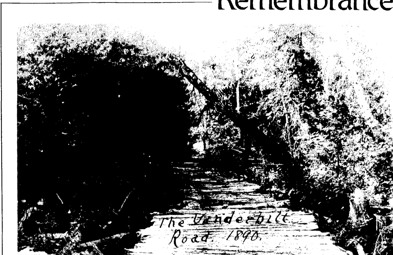
Back in 1890 the road to Vanderbilt had many areas where planking was used through the swamps. This picture shows one of those areas. Many of the roads in Northern Michigan
