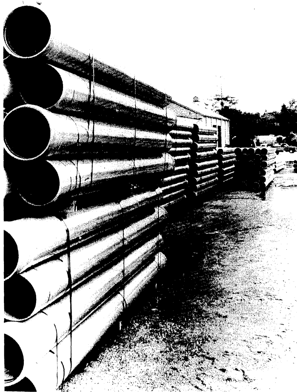
Pipes are ready to go into the ground, after they have been displayed in Boyne City's Veterans Park while waiting to be taken to where the new water lines will be installed along many of the streets during the rebuilding of the city's infrastructure. Although the pipes are different colors, the green and the blue will be used for water mains. The black pipe will be fused together as part of the slip lining on the sanitary sewer along Lake Street.
