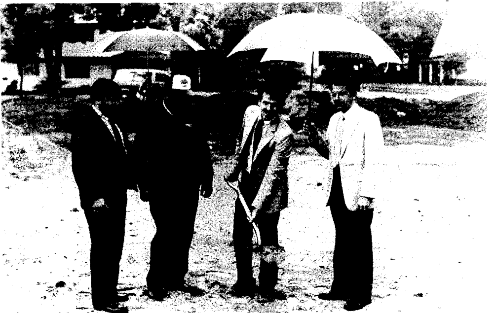
Turning over the first shovel at their rain soaked ground breaking for the new Burns Clinic is Dr. Alan Fark, one of the staff who will be headquartered in the new building. Holding the umbrellas while they watch are Bob Crumb, assistant administrator of the clinic; Tom Garlock, representing the City of Boyne
