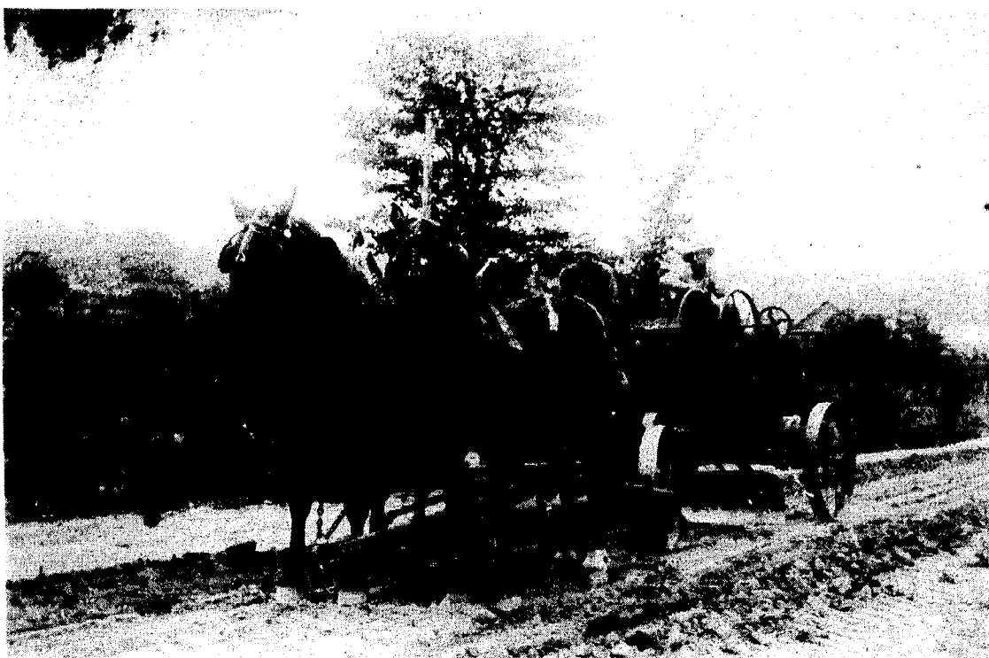
It took about a day to grade a mile of freshly laid gravel road as this team of horses pulled a grader during the making of the road that goes to Horton Bay. The horse crew would go back and forth along the road until they spread out the
