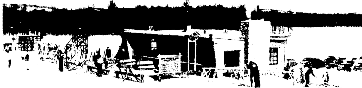
BOYNE MOUNTAIN LODGE Boyne Falls, Michigan
