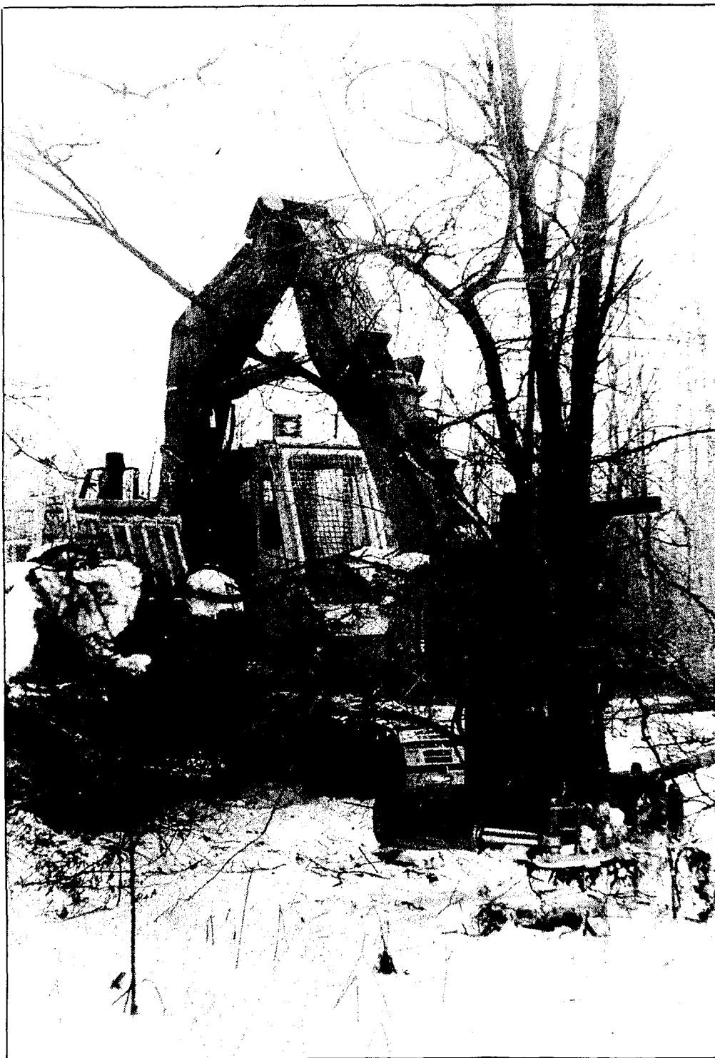
Lumbering came to Boyne City last week when thinning and lumbering started in Boyne's Rotary Park. The heavy equipment came in and clipped out all of the trees marked by area foresters. The trees were then piled awaiting a chipper which will
