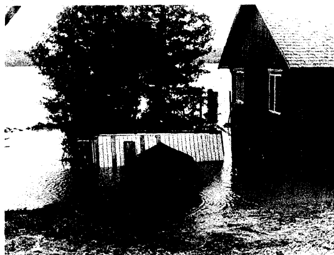
One of the cottages next to the lake along the road to Advance found about eight inches of water covering the lawn and flooding out the well house.
