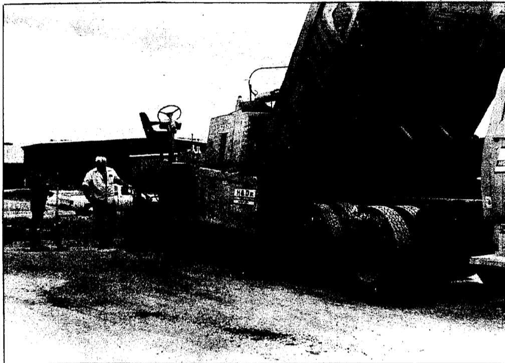
Workers from Hodgekiss and Douma started to lay the asphalt on the roads of the new Air/Industrial Park Tuesday. The pavement will be ready for driving upon this weekend, according to officials from the firm. The asphalt is being laid in two lifts of three inches each to provide a heavy duty surface for the many heavy trucks which are expected to be using the roads.
