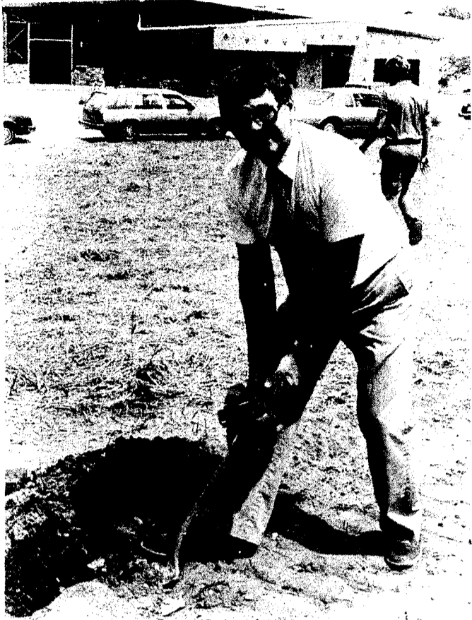
Doug Shields turns a spade of dirt to signify the ground breaking for his new home for the Prestige Press. The 4,800 sq. ft. building is the first building going into the new industrial park located on the outskirts of Boyne City. Shields expects to be in the building by the end of November. Also breaking ground last week is the new building for Temprel Products Company. They will be located across the street from Prestige Press.
