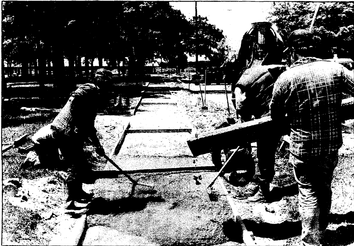
The beginning of a long pouring of cement started Tuesday as workers started to fill the new sidewalk forms at the Old City Park with cement. The crew from the O.D. Sayles Masonry won the bid last week and have finished the job in time for the first weekend of the Farmers' Market
