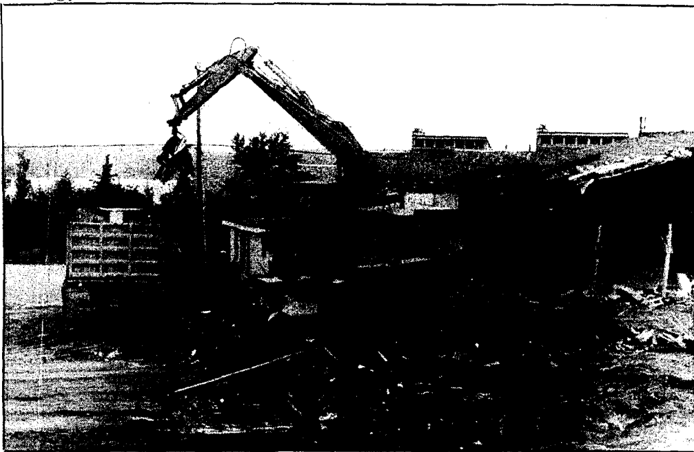
Tearing down the old Boyne City Locker Plant along North Lake Street was a crew from Dunkel Excavating. The proposed plan would involve the changing of zoning for the land from general business to multiple dwelling. A public hearing is slated for the change down to make room for a proposed condominium project.
