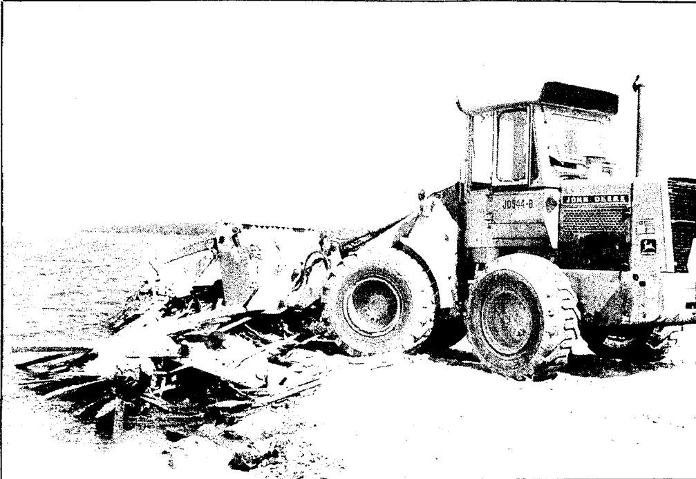
If you're looking for a source of firewood for next winter, see the workers building the new municipal beach. They ran into a mess of slab wood that has been buried in the lake since the lumbering days. Here workers are taking the slab wood to a site to have it burned.
