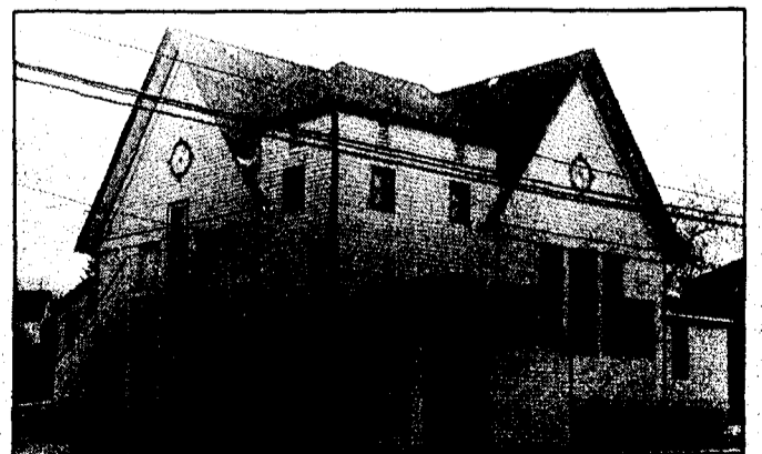
Under consideration as the future Boyne City Museum, this structure, located across the street from the Charlevoix County Press was recommended for purchase by the city's historical commission. The city is going to have to make the purchase, and city commissioners were asked to look through the structure which was built in the early 1900's as the Baptist Church, to make sure it would fit the city's needs.
