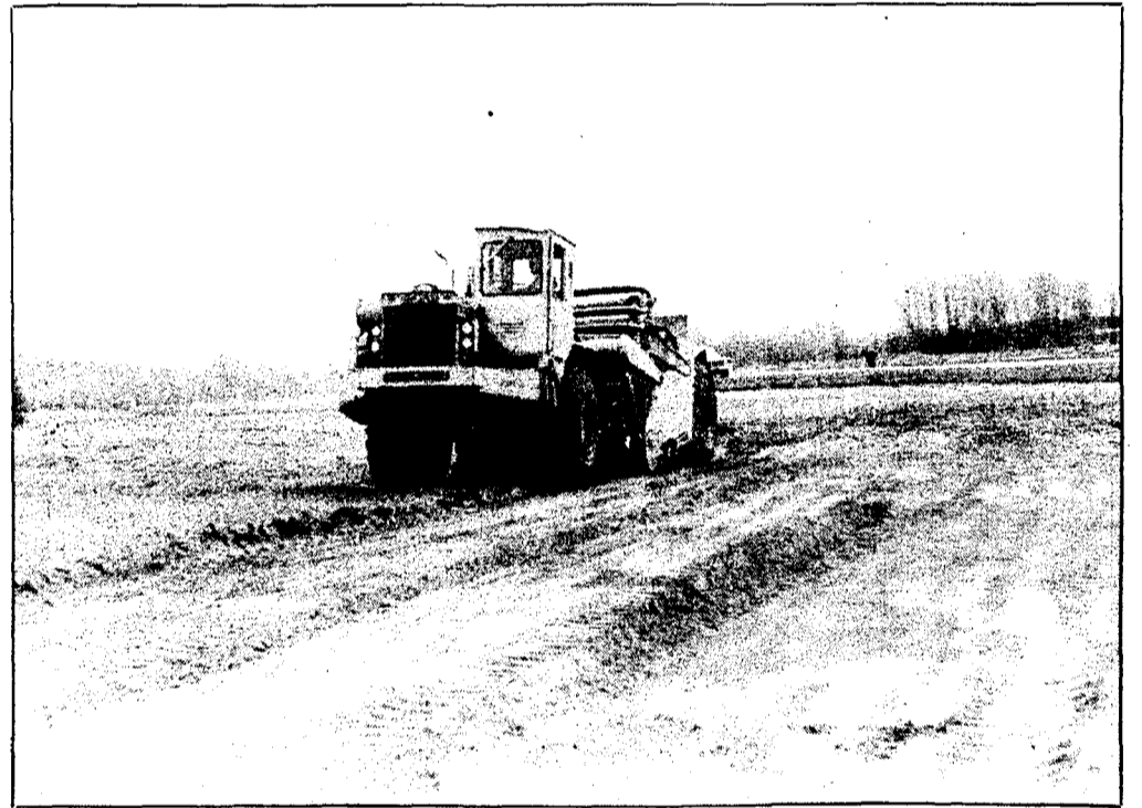
Earth movers started the preliminary work to extend the runway at the Boyne City Airport Tuesday. Hodgekiss and Douma won the bid for the extension
