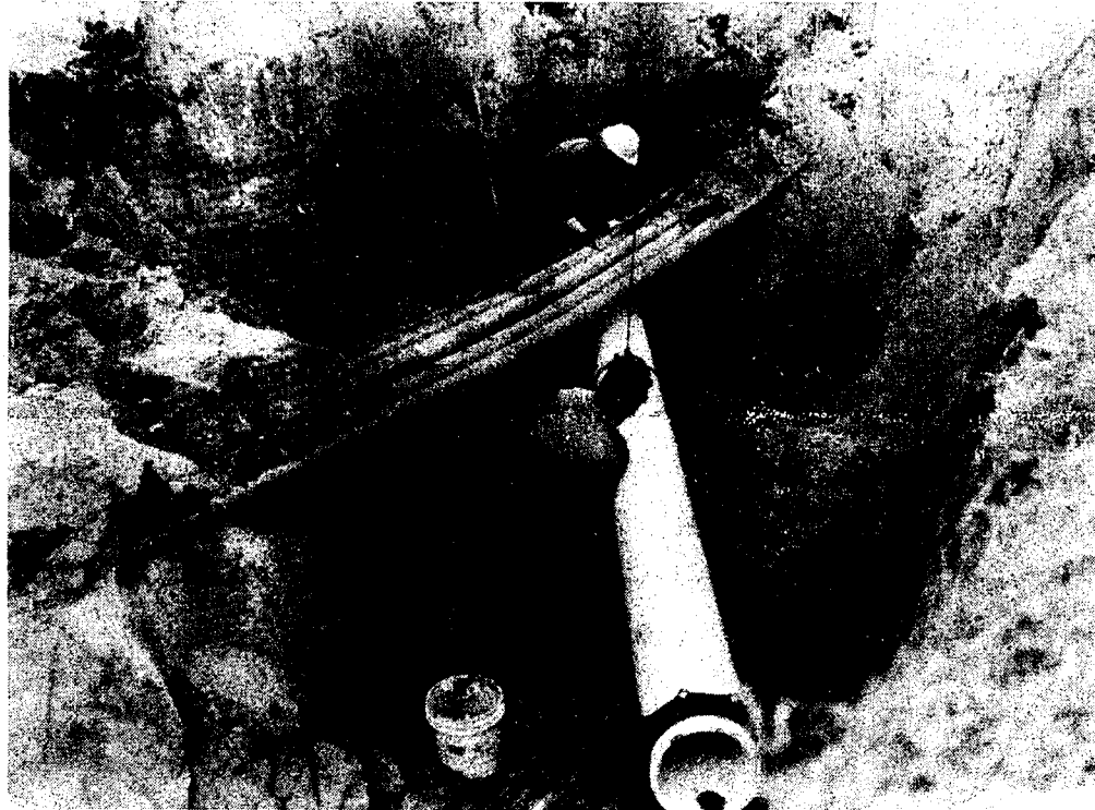
Water main work along Division Street is progressing nicely as crews from the C.H. Smith and Company work towards the new Air/Industrial Park. The watermain will serve the park and will provide looped service for other neighborhoods in the area of the airport.
