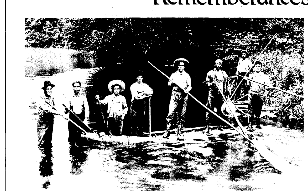
Along about this time of year, with the advent of high water on the rivers and lakes, men with canthook and peevy would have the wet and hazardous job of riding logs down rivers to mills. A notation on this old picture says, "We have watched them jockey a boom of logs being towed through the channel to the Charlevoix Lumber Co."
