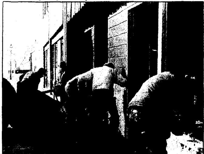
With the break in the weather, the workmen remodeling the old Lil Pub into a new pizzeria broke out the exterior walls to get them ready for the new glass. The work is being done by Jim Daniels Carpentry along with help from the owners of Little Lena's who will be utilizing the new location. The restaurant will be featuring table service as well as the continuation of the takeout business.
