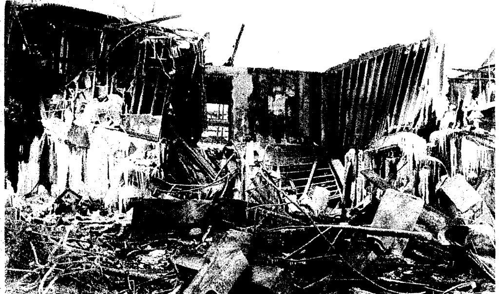
The next day, the rubble of the fire was squirting water from the many water pipes that had melted from the intense heat. Insurance inspectors and officers from the State Fire Marshall's office will make the determination as to the cause of the New Year's Eve fire.
