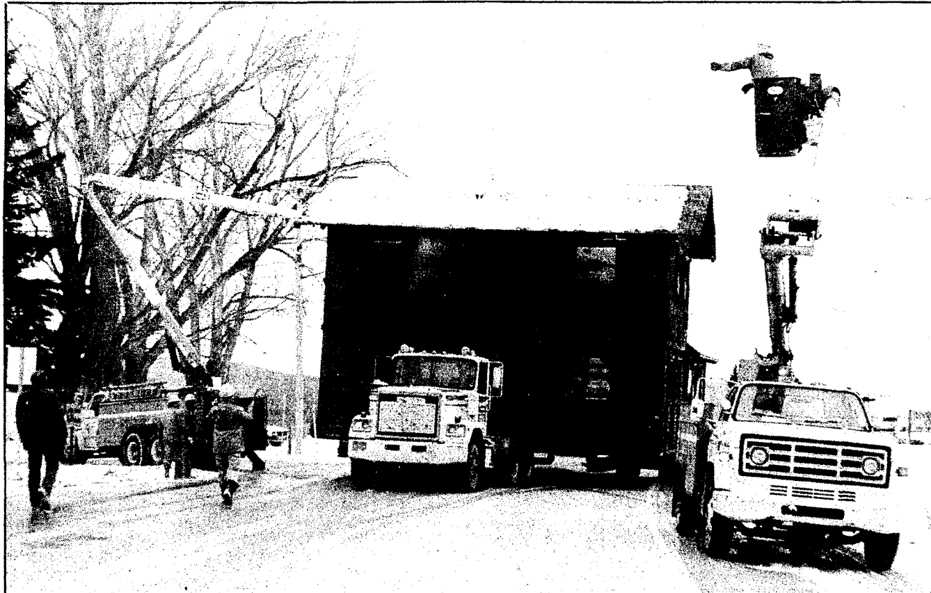
Moving a house creates all kinds of excitement. Last Monday, one of the Boyne Falls Log Homes was moved from Boyne Falls to a site on Hayden's Pointe next to Whiting Park. The move required the hopscotching efforts of Consumers Power, Wolverine Power, Top O'Michigan, and the cable company as the building went down the road to its new home. The building
