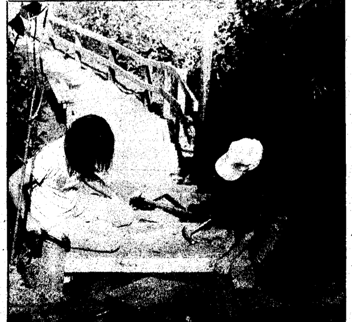
Lisa Amesbury and Maria Baker, both of Boyne City install steps on a path down to Lake Michigan at the Townline project. Seeding and landscaping was also done at the site.
