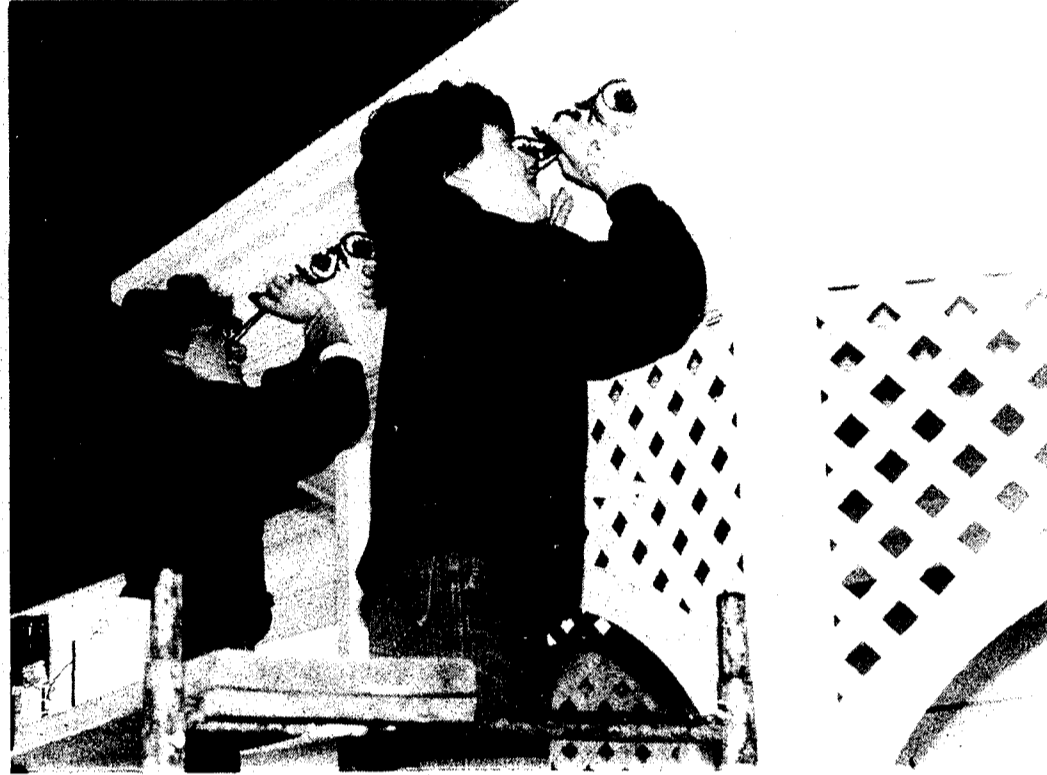
Art students from Boyne City High School art classes were hired by the contractor who is building Stafford's One Water Street Restaurant to paint some of the detailed art along a cornice that is being built in the main
