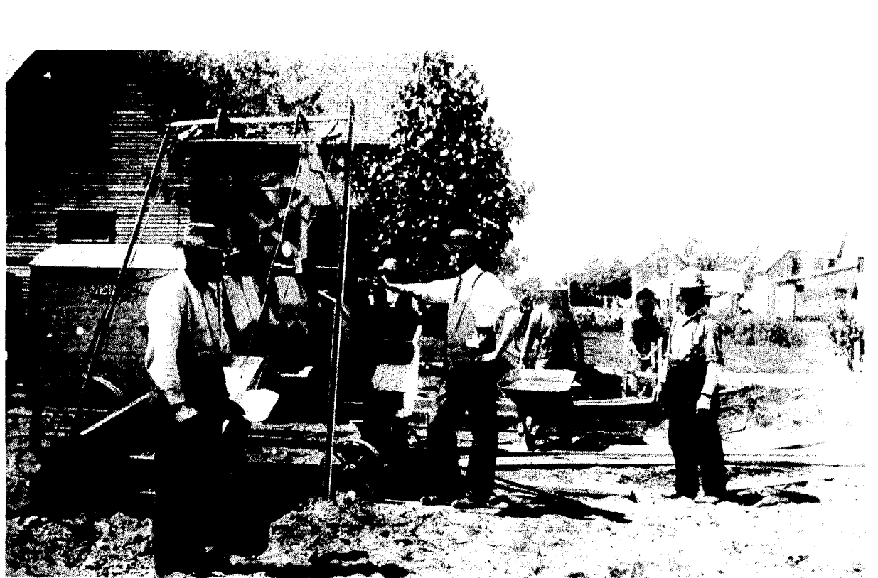
Back when the streets were first being installed in Boyne City, this crew went out to make the curbs and gutters with their equipment. We don't know whether the man at the cement mixer wore what looks like his Sunday best everyday, or if it was just for this picture.
