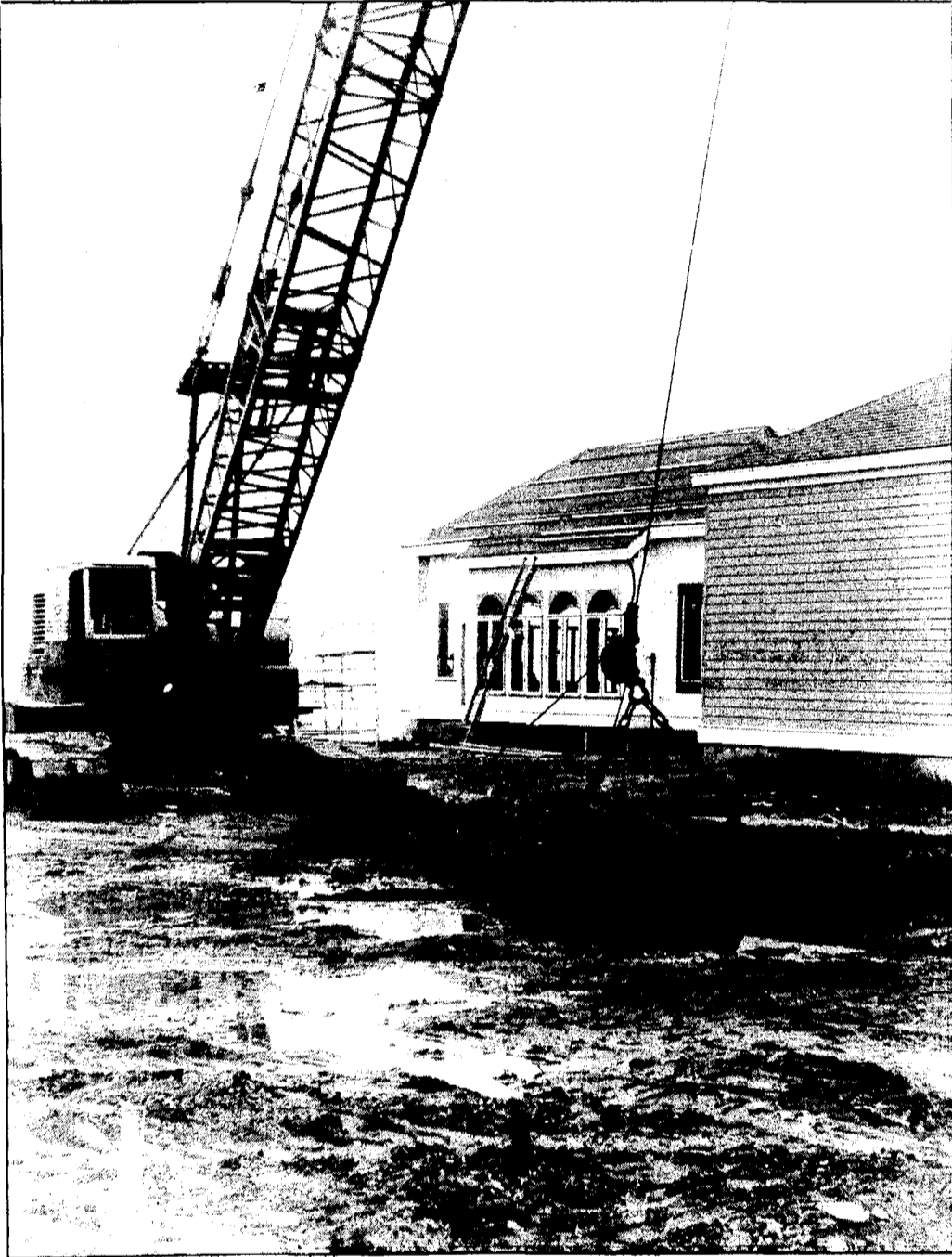
Digging for the moat that will surround the new Stafford's One Water Street Restaurant was started Monday. The dragline of C.H. Smith and Company is performing the work of digging out the channel that will separate the restaurant from the land. The company had to dig through layers of slab wood that was used as fill when the lumber and railroad companies moved into the land back at the turn of the century.
