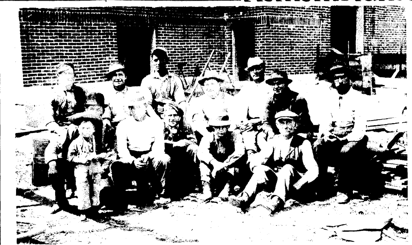
This picture shows the construction crew that built the Wolverine Hotel in Boyne City. The hotel is now known as the Dilworth and is still standing, awaiting conversion to a bed and breakfast hotel. The building was one of the first projects of the Price Bros. Construction firm which is still in existence but known as Price Bros. Marine Construction Company located in Ohio. They have grown to be one of the largest in the field according to Bill Underhill, who supplied us
