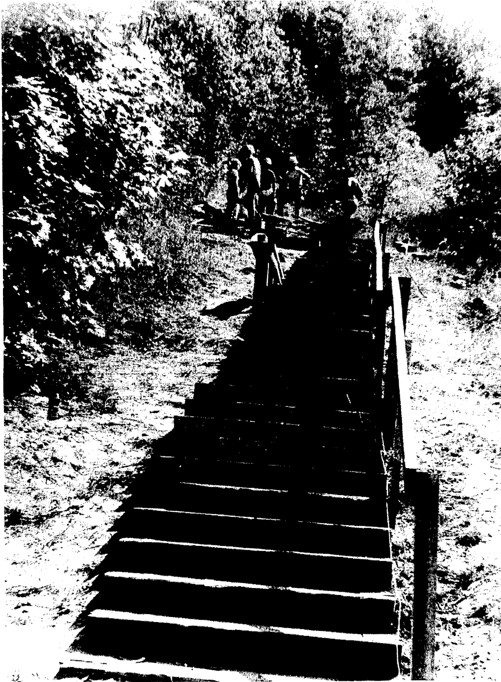
Youth corps workers are slowly making their way up the hill in the Avalanche Preserve, building steps as they go. The steps will allow sight seers access to the top for the view of the Boyne City, Lake Charlevoix area. Every few
