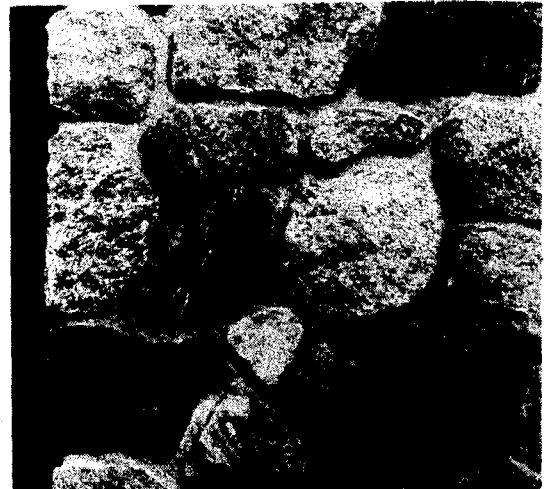
For his own house, stonemason Hans Kretschmann used cut stone set in mortar that is, as the layman might say, indented, giving the stones more emphasis.
