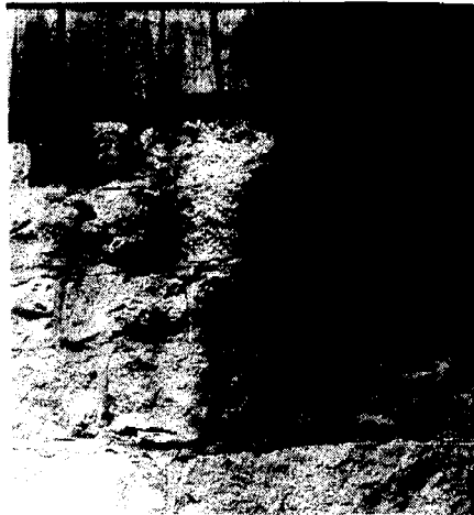
Painstakingly cut into block shapes, gray, pink, and green stones make a strong foundation for this fine barn, built by the Pesek brothers near East Jordan.
