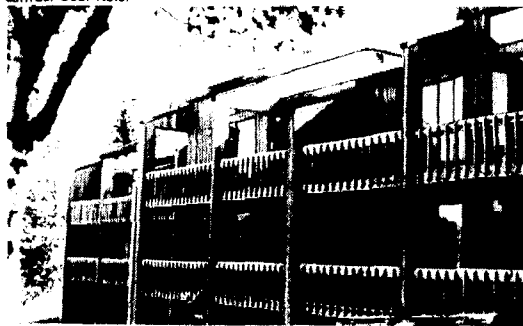
Located on the Pine River Channel, which connects Lake Michigan with Round Lake Harbor. This two bedroom, full furnished unit offers significant living, low maintenance, convenient rental opportunities, and just one block from the unique downtown Charlevoix shops. Call Suzi Reis today for further details.
