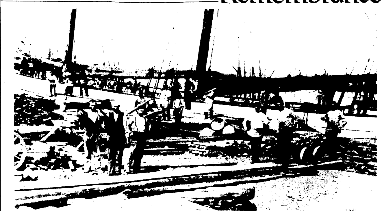
Loading pig iron was one of the summertime jobs for many men at the Ironton Pig Iron Company as well as the foundry in Boyne City. The pigs, as they were called, of cast iron were loaded onto trolleys and pushed down to the boat where they were manhandled onto the ship for distant points. This ship was one of the many schooners that plied the Great
