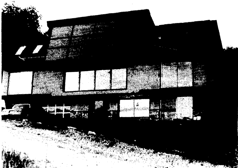
The house of Betty and David Korthase is almost as marvelous for its views as for its solar heating. Korthase backs it with a wood stove and, for while they are away, with electric heat.
