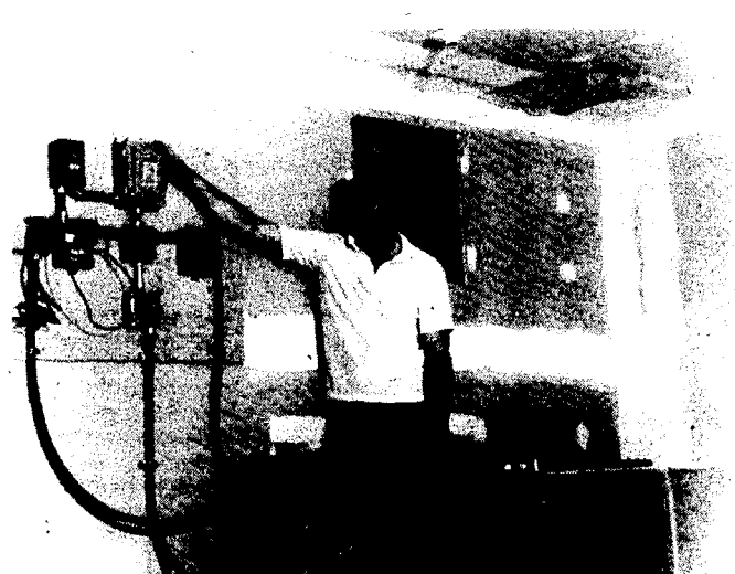
David Korthase's hand is on the controls in the solar house he designed and built. He stands behind the series of storage boxes containing, at the moment, 132 degrees of solar heat. The controls turn the fan on and off, keeping the house in the pleasant low 70s.
