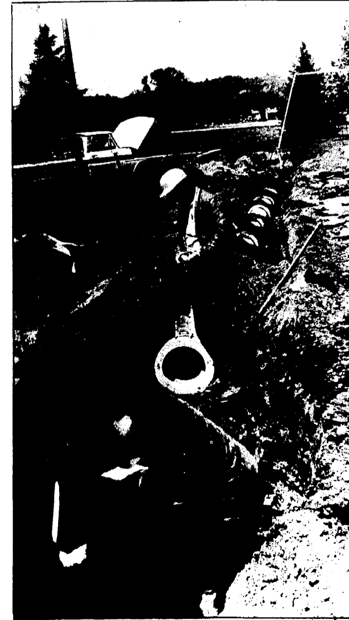
Work is progressing slowly on the Front Street extension as the workers from the C.R. Smith Company finish up the laying of the storm sewer along the roadway. The workers will be laying the water mains and doing the construction for the sanitary sewer before adding fill gravel and building the curbing. Work is expected to be finished prior to the Fourth of July.
